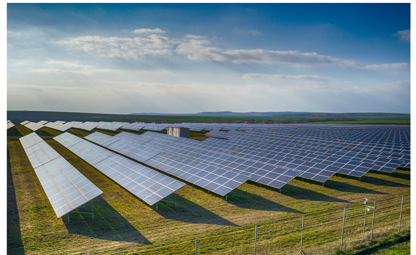
Example of Solar Arrays on Solar Farm
